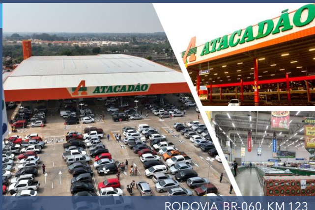
RODOVIA BR-060, KM 123
