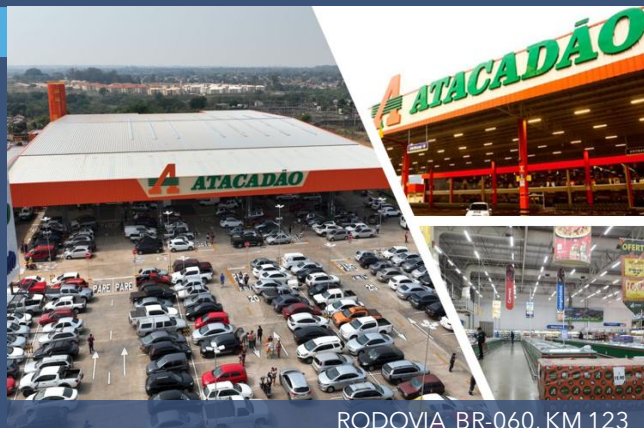
RODOVIA BR-060, KM 123
